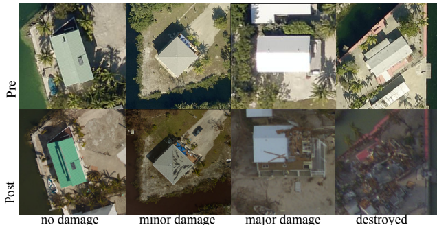
Figure 1. Samples of aerial photographs depicting the different levels of damage caused by Hurricane Irma on the Florida Keys.
